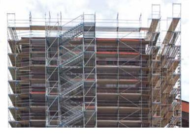
The concept of the Scafom-rux universal stair tower is based on a 12- to 24-leg scaffold base and meets the increased requirements resulting from the German Regulations on Places of Assembly.
